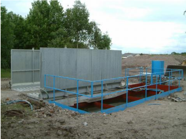
FORCE SIX WASH DECK WITH 44m 3 STEEL IN-GROUND RECYCLING TANK
