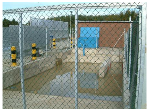
FORCE SIX WASH DECK WITH CONCRETE DECANTATION PIT AND RAMPED LOADER ACCESS FOR SPOIL REMOVAL
