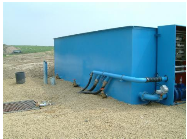
FORCE SIX WASH DECK WITH 38m 3 STEEL ABOVE GROUND RECYCLING
