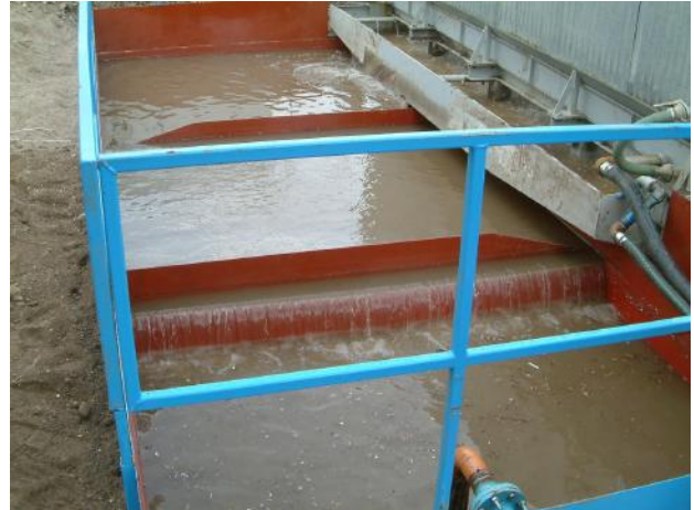
FORCE SIX WASH DECK WITH 44m 3 STEEL IN-GROUND RECYCLING TANK
